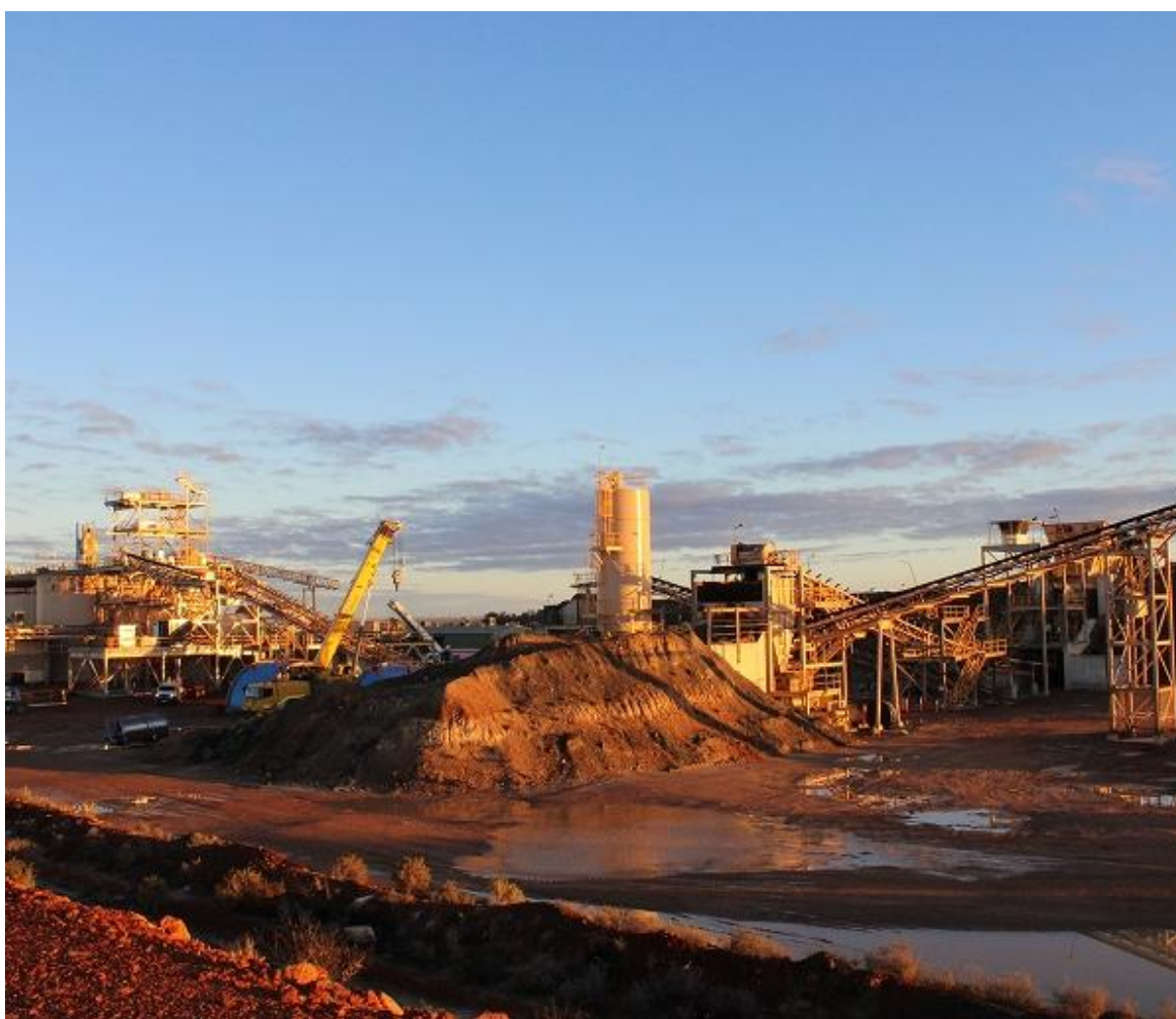
Figure 2. Kirkalocka Gold Processing Plant (operated by Gylden Resources Pty Ltd)
