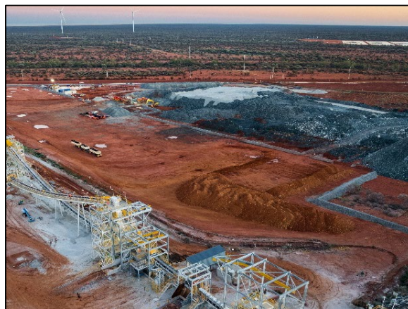
Figure 8: Waste rock crushing and earthworks for permanent Mine Services Area
