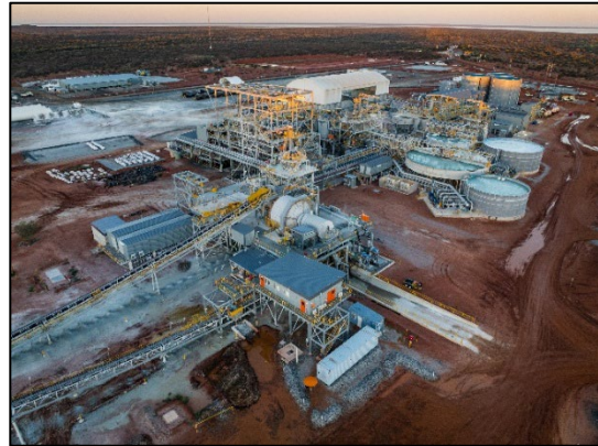
Figure 4: Aerial view of process plant
