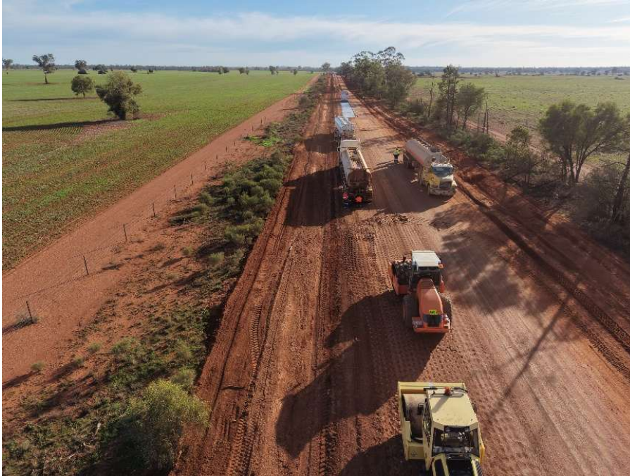
Figure 3: Constellation haul road construction
