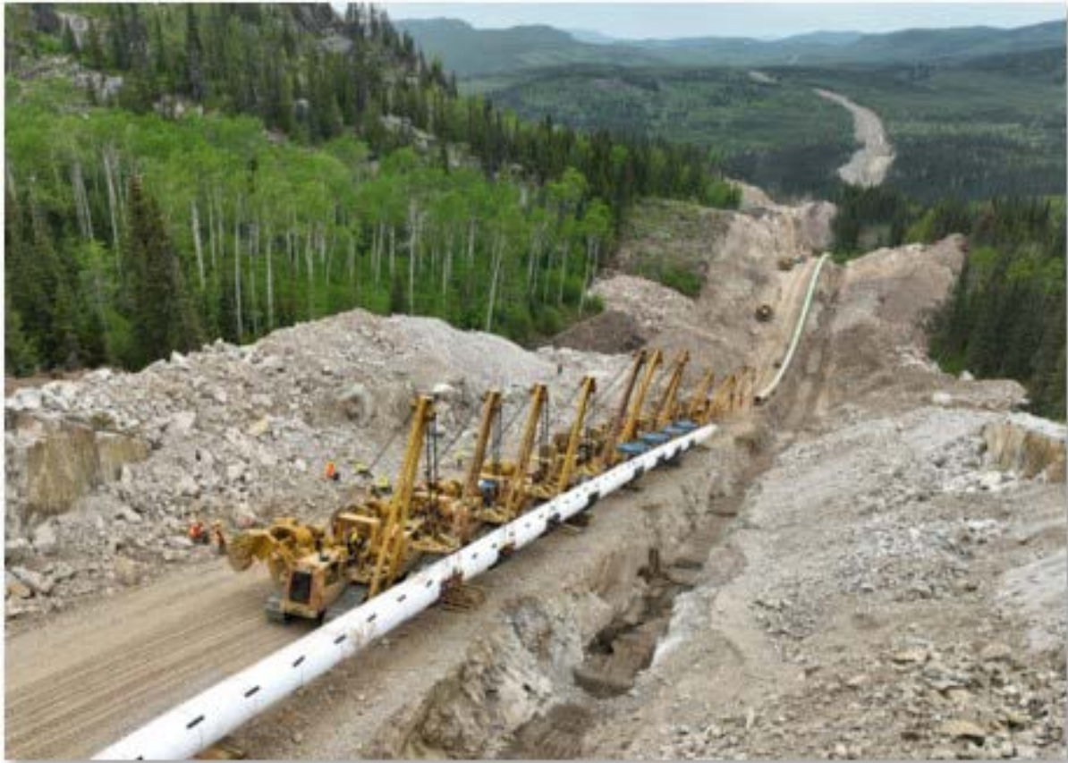
Figure 26: Typical pipeline installation site works. Courtesy Fortin Pipelines.
