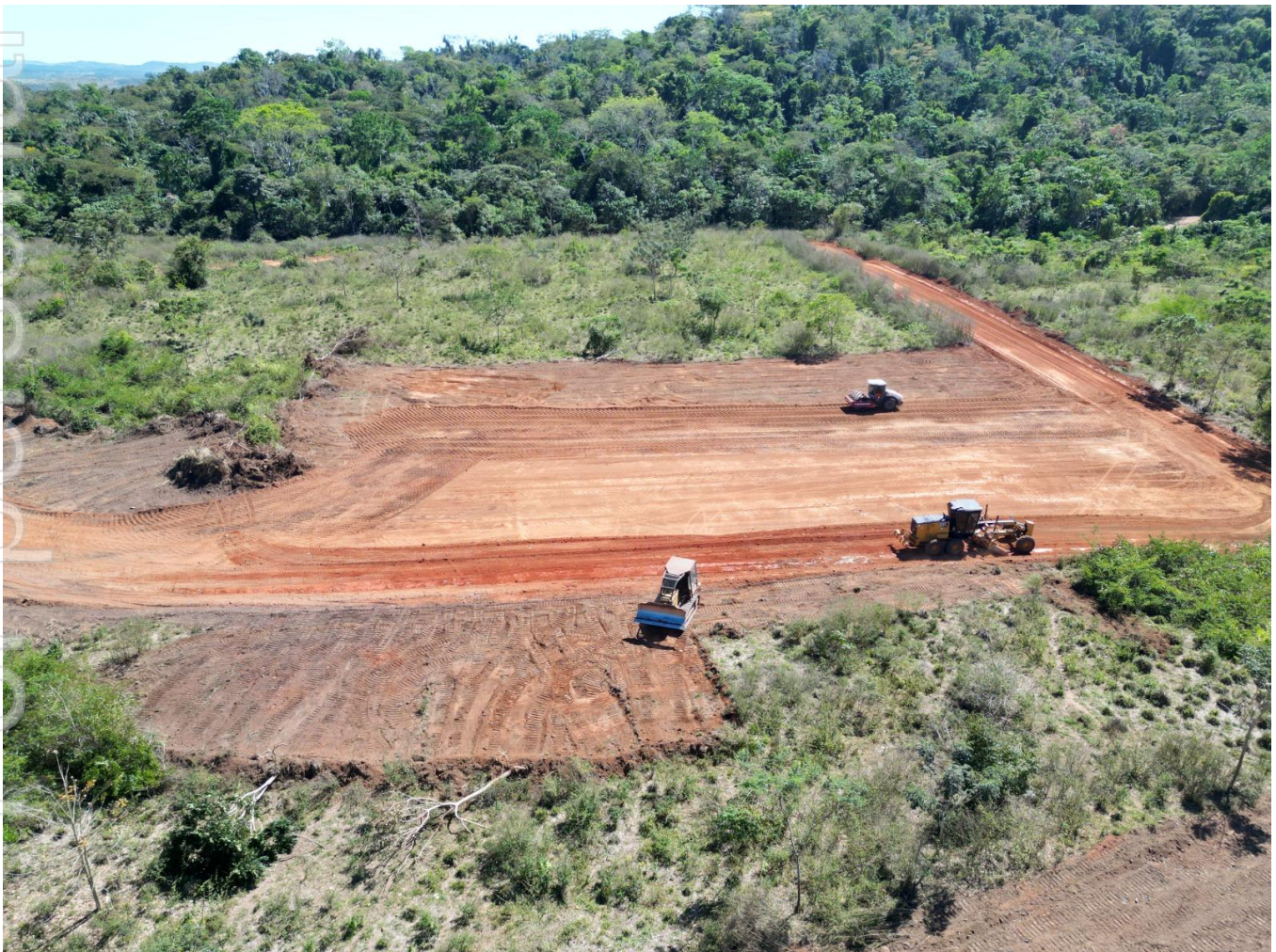
Figure 2 – Jaguar Project Pre-Development Earthworks
