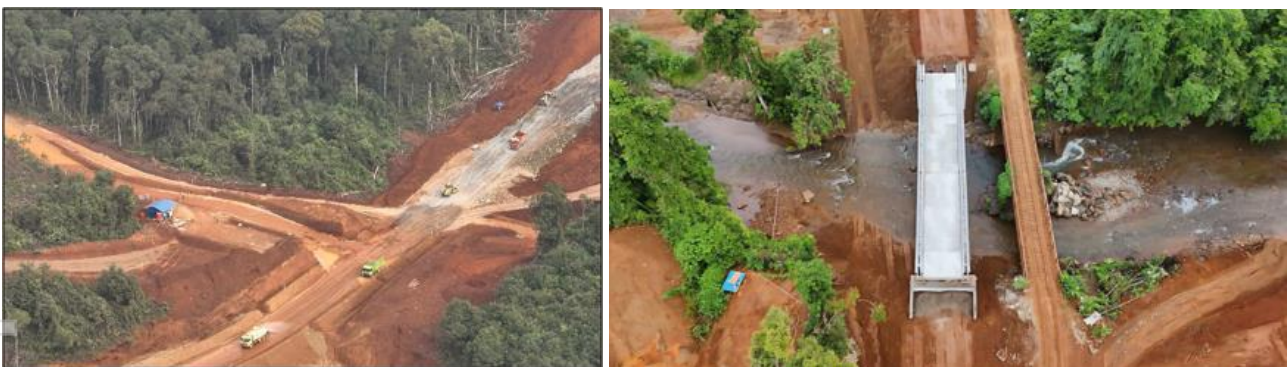
Sampala Mine construction activities
