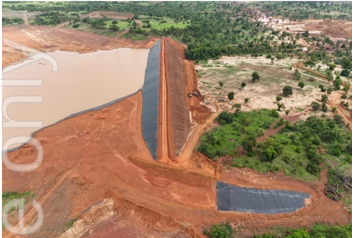
Figure 7: Water Storage Dam - Lined Spillway and Embankment
