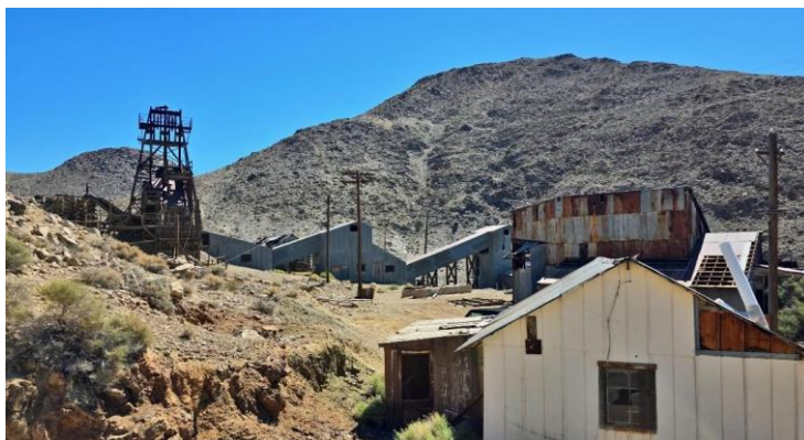
Figure 1: Nevada Scheelite Mine headframe, mill buildings and surface infrastructure, looking northeast.
