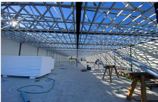
Progress at permanent Mine Services Area (MSA)
