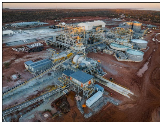
Figure 4: Aerial view of process plant
