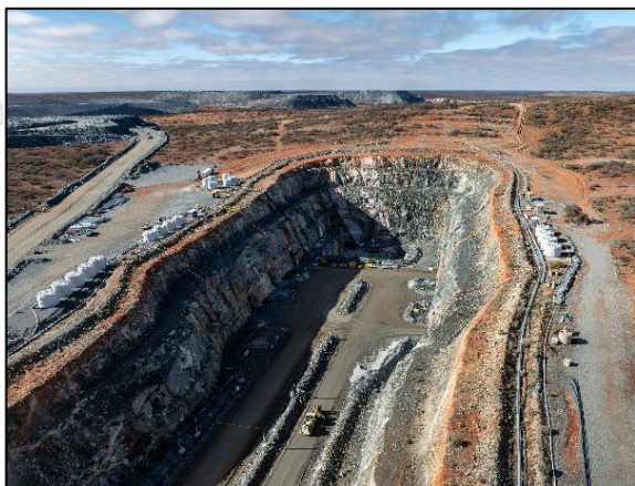
Figure 7: Infrastructure preparation at North-West Flats
