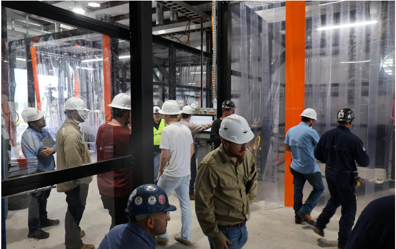
Figure 4: Our primary reactor test building contains four commercial-scale semi-batch FJH reactors
