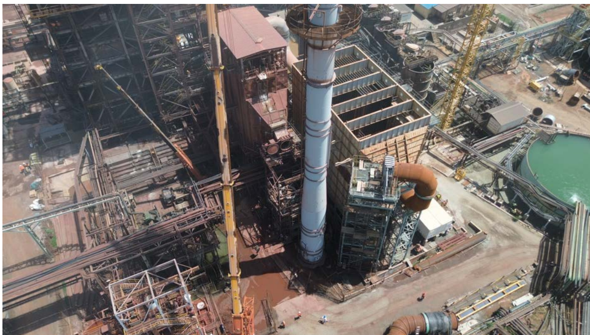
Figure 8: New Electrostatic Precipitator being tied in
