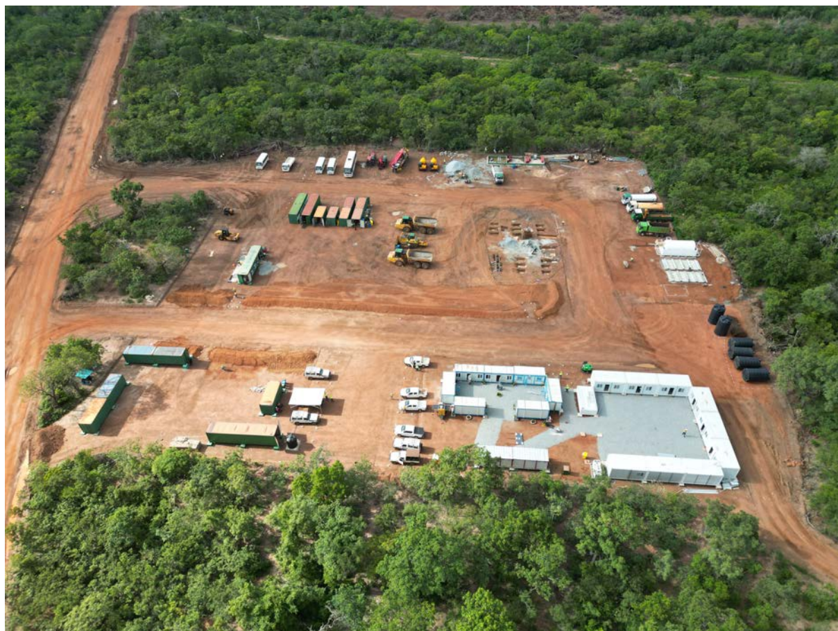
Figure 3: Contractor Laydown and Resolute Construction Offices
