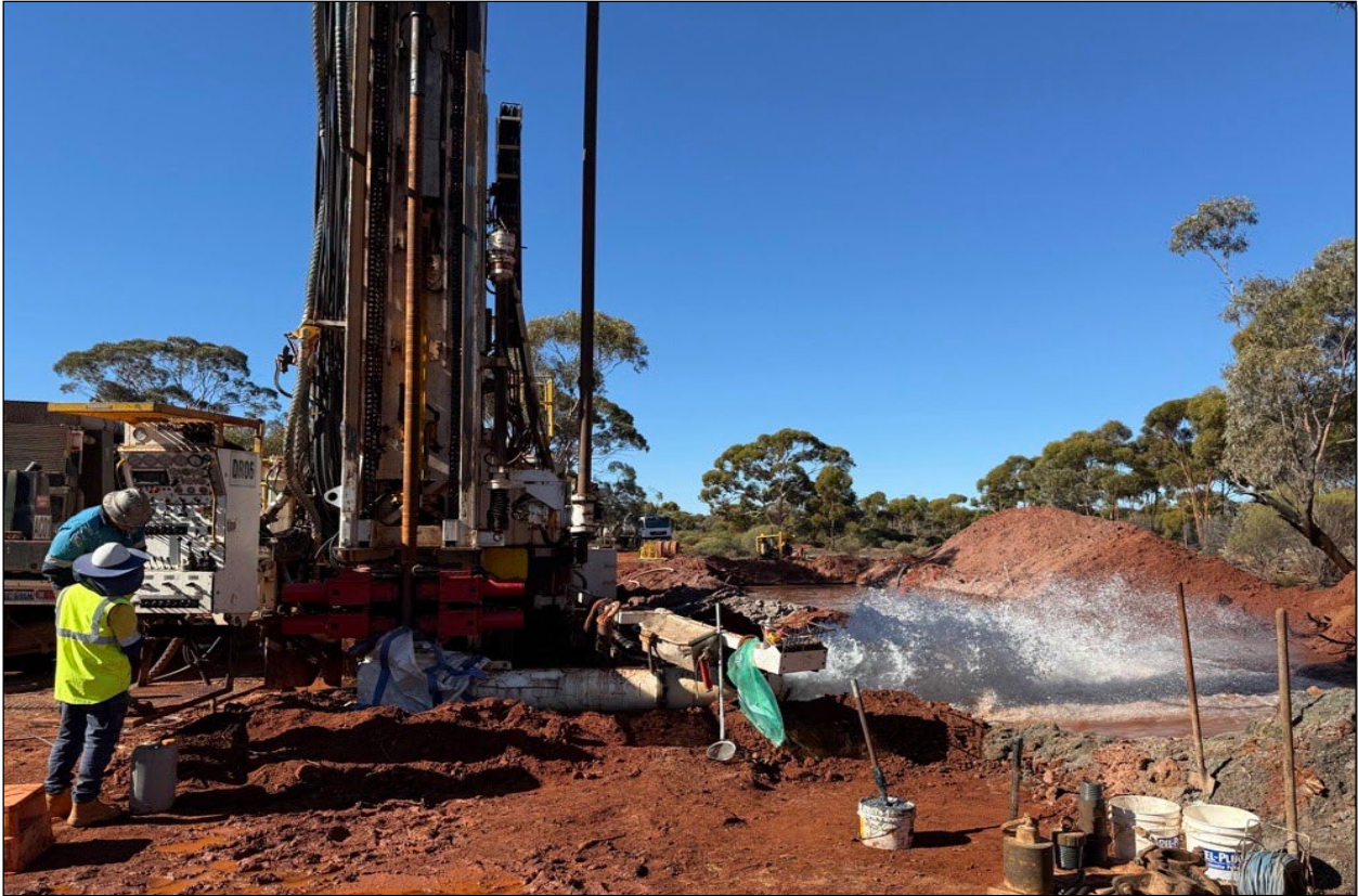
Figure 4: Water bore airlift testing and installation
