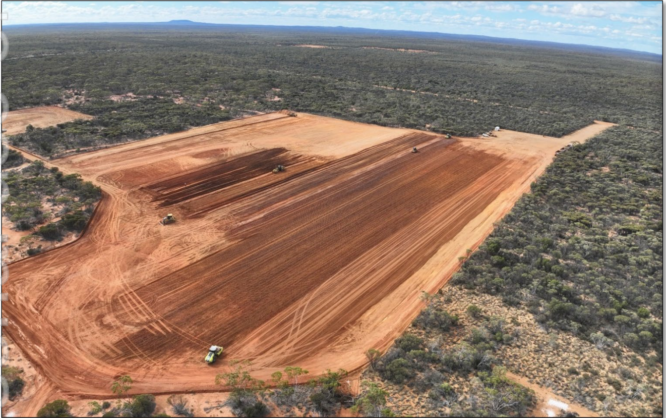
Figure 2: Bulk earthworks for the accommodation village
