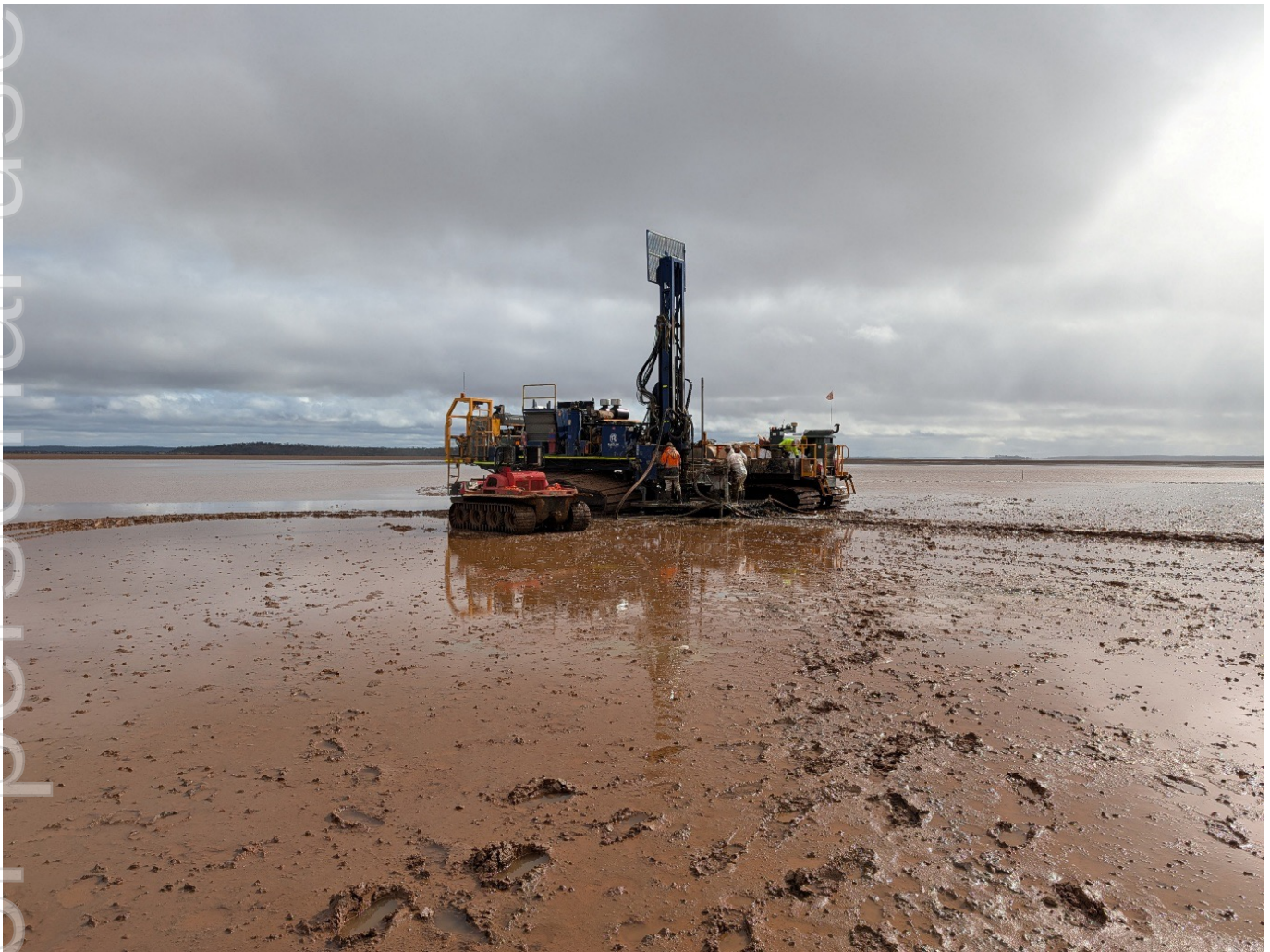
Photo: Drilling Underway at Lake Cowan.
