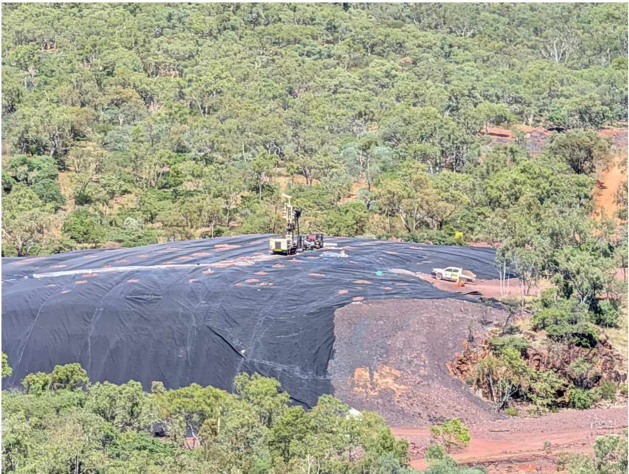
Figure 6 . Sonic drilling rig conducting a characterisation drill program on a legacy mine materials stockpile at Mount Oxide.
