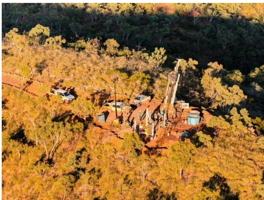
Figure 4: Drill Rig onsite at Mt Oxide during the Quarter
