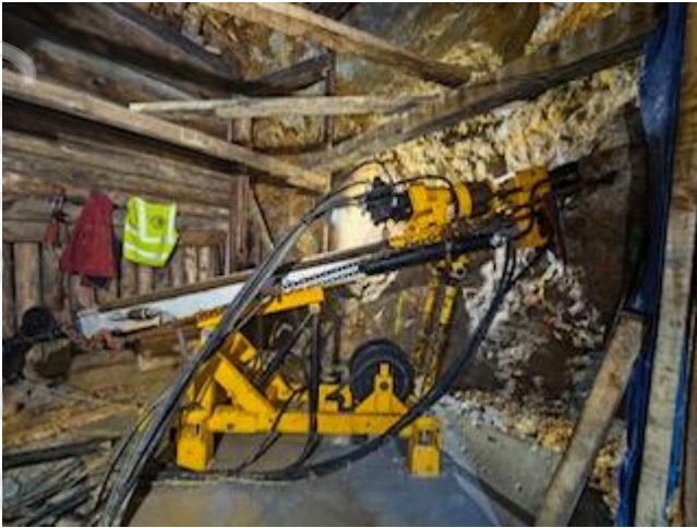
Fig 1: Drilling first 5 holes from Chamber One
