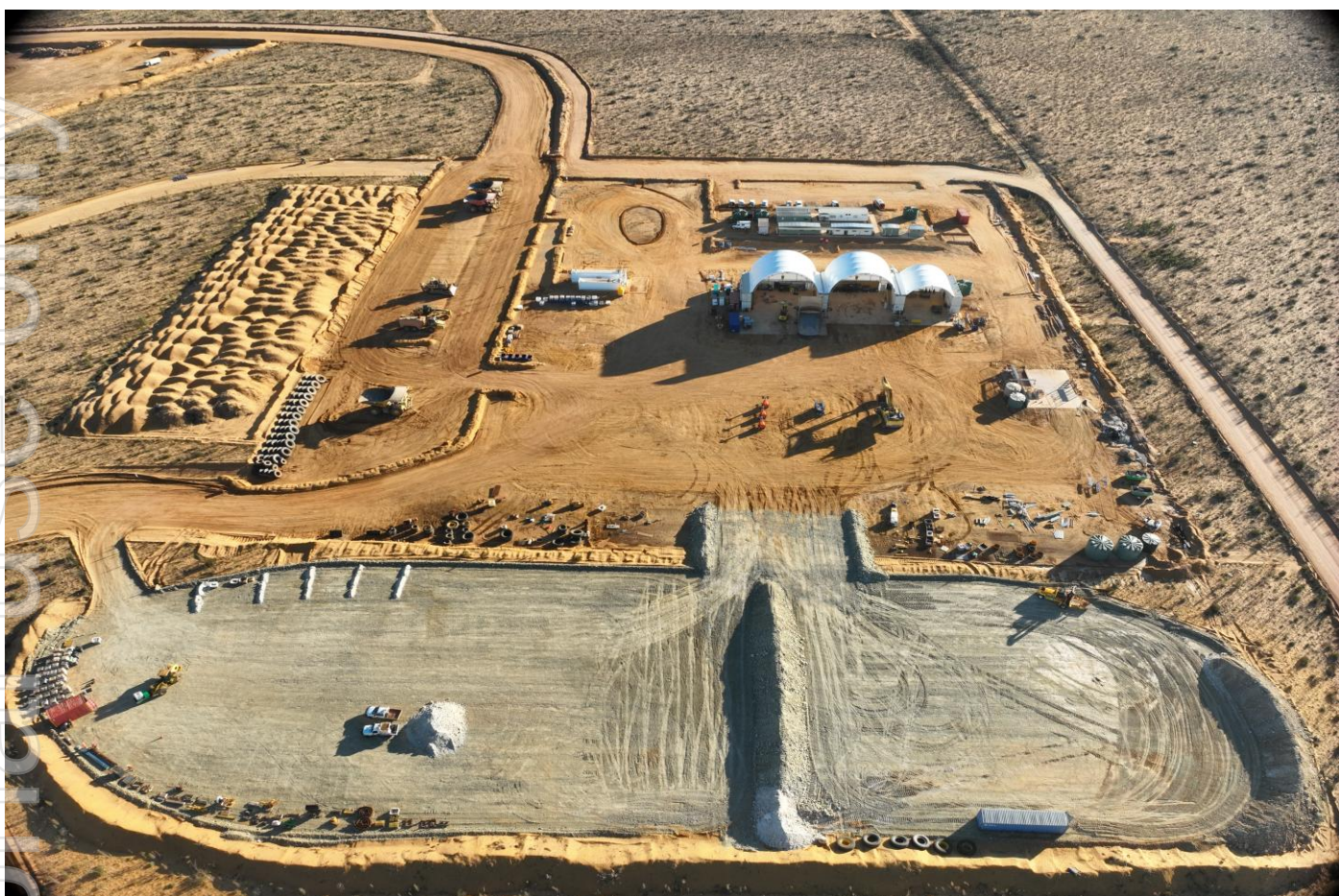
Image 2: Workshops, Offices and Infrastructure at Iguana 28 July 2026
