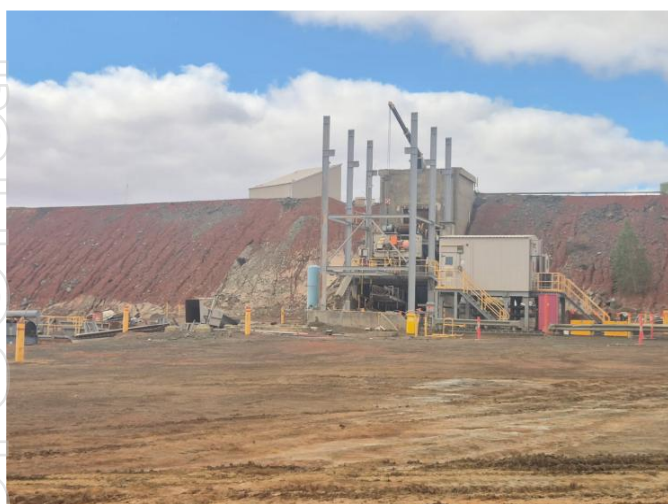
Figure 1: Primary Crusher Conveyor Removed
