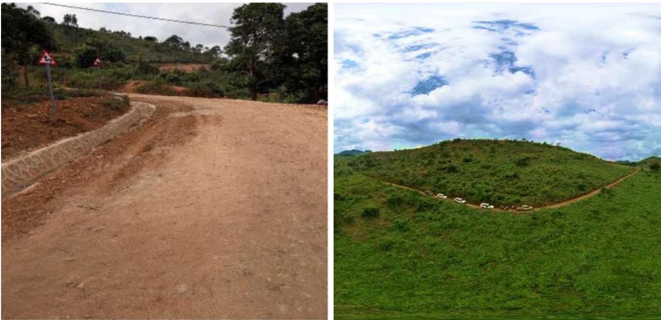
Figure 1 – Southern Access Road
