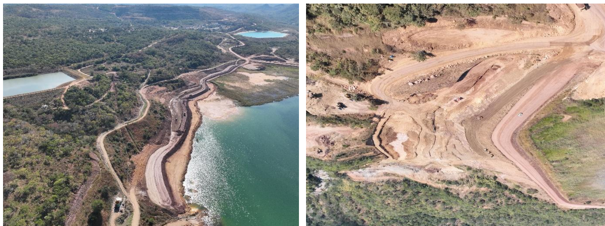
Figures 3 and 4: TSF expansion works, June 2026
