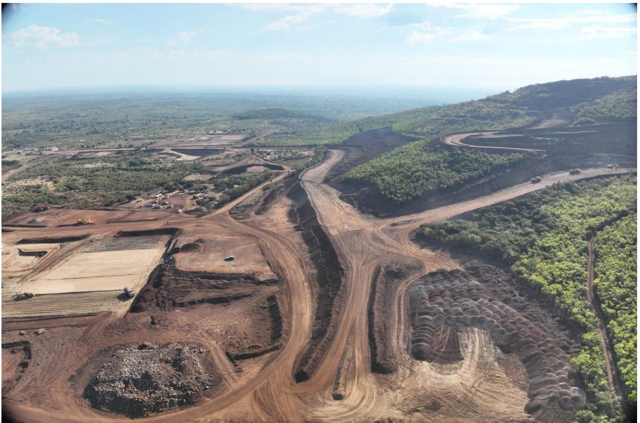
Picture 6. ROM pad and mining skyway
