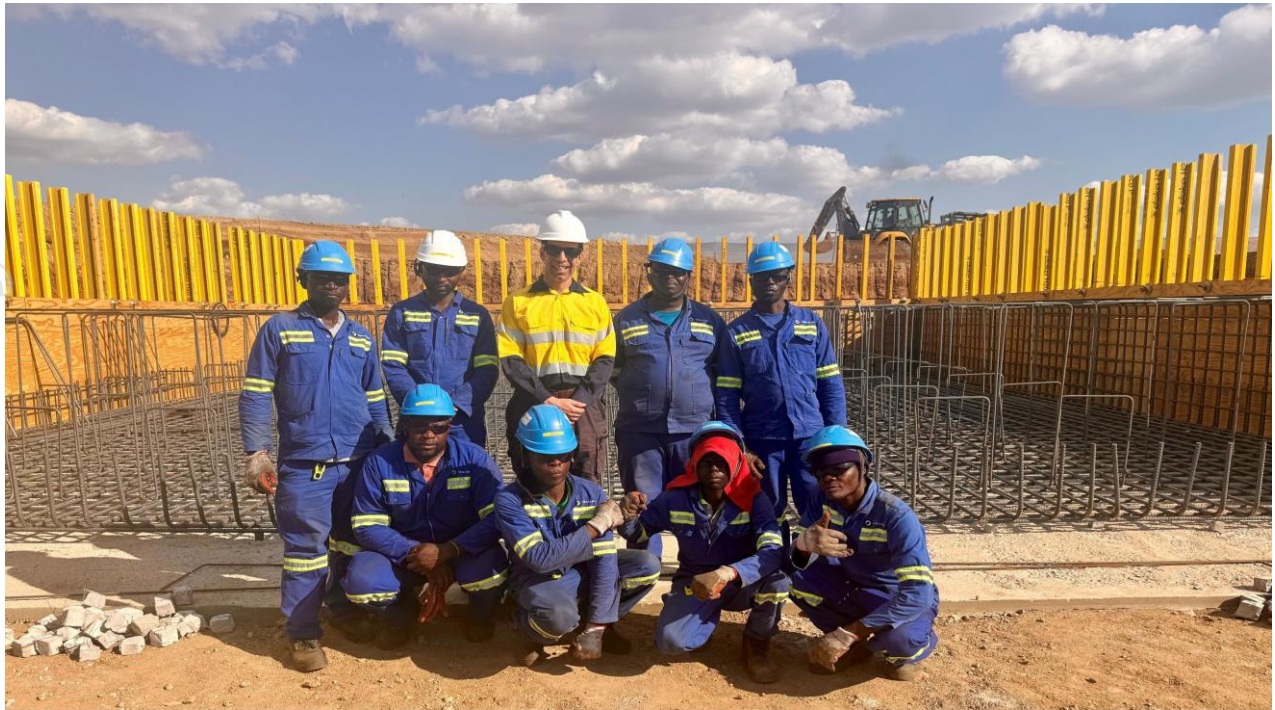
Picture 1. Lindian Resources Executive Director Zac Komur with the Kangankunde construction team at the SAG mill foundation area, where process plant civil works continue to advance
