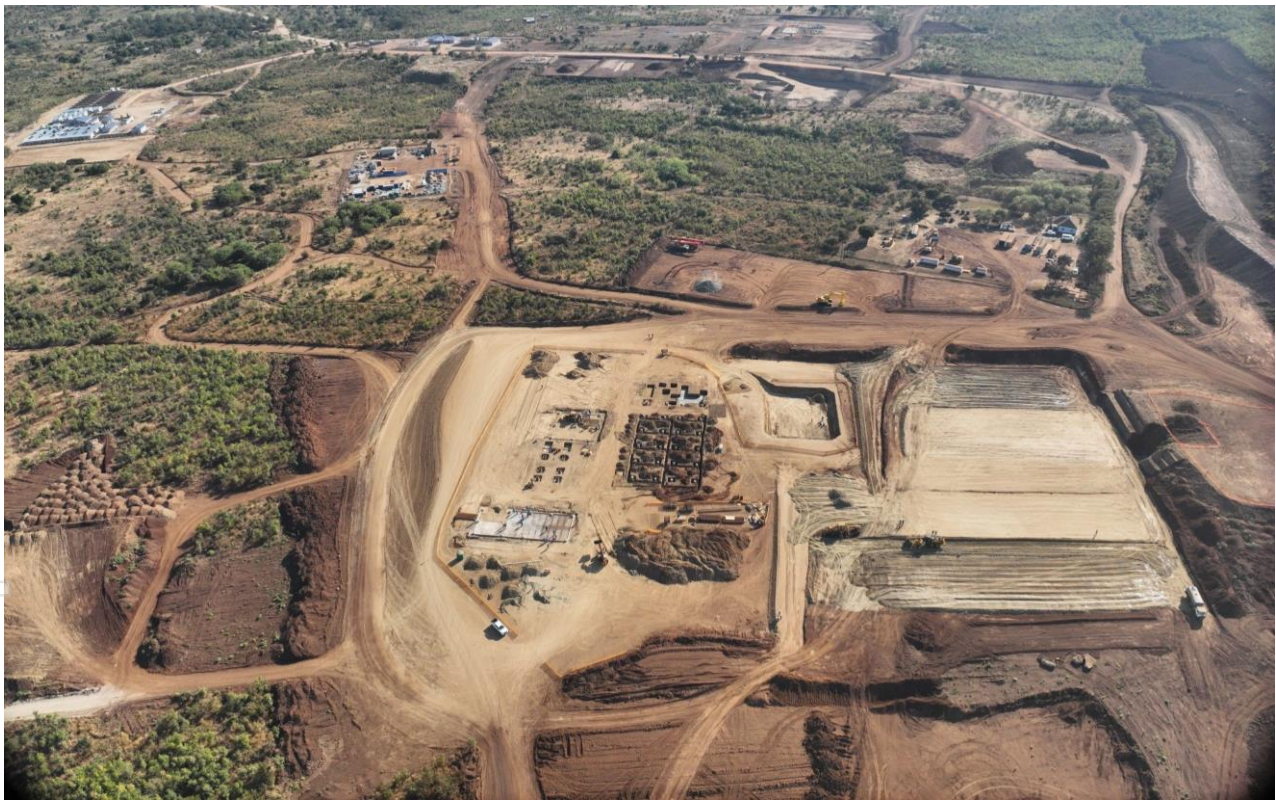
Picture 2. Overview of the Kangankunde process plant area, highlighting continued progress across civil works, earthworks and supporting infrastructure
