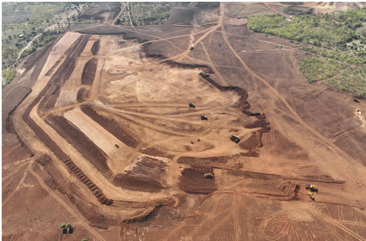
Picture 8. Kangankunde Tailings Storage Facility Progress
