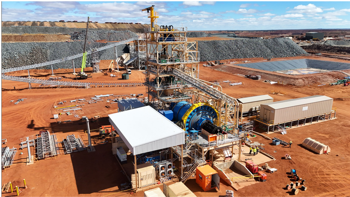
Karlawinda Expansion Project – Mill area nearing completion.
