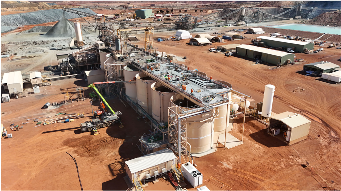
Karlawinda Expansion Project – CIL circuit extension with top of tank steel sections in place.
