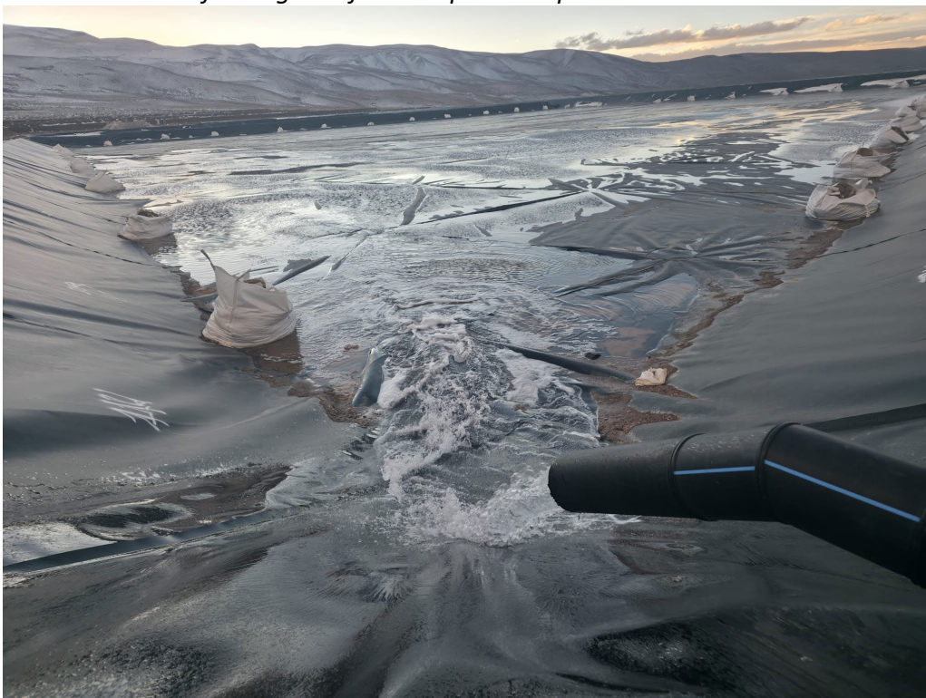
Figure 3. Processed brine flowing into final evaporation pond.
