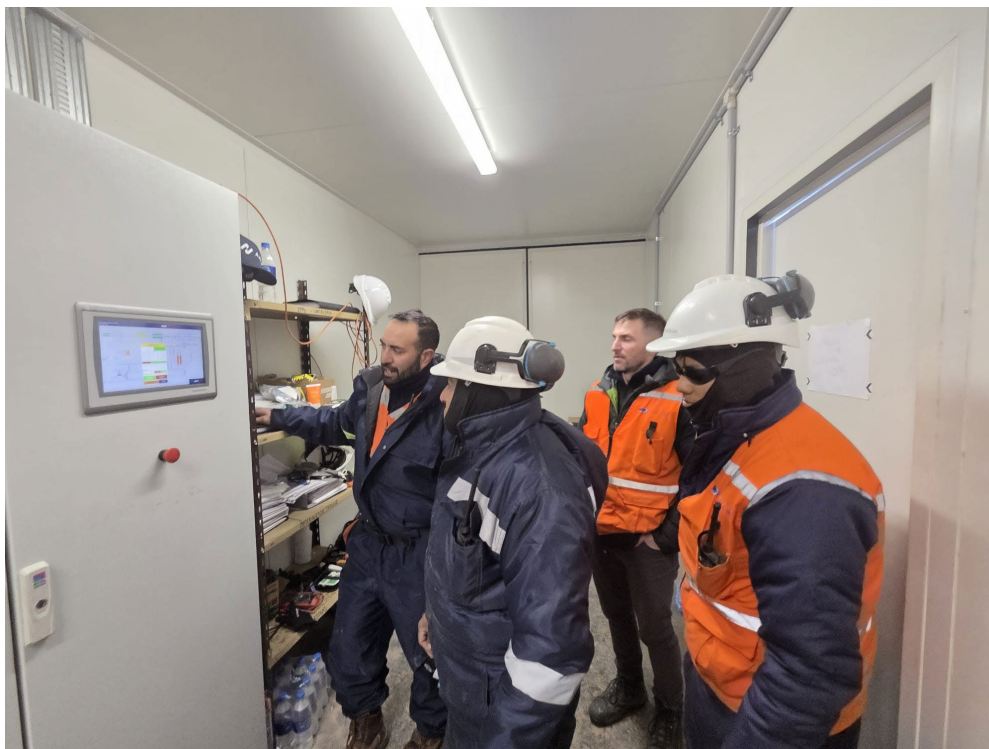
Figure 5. Operators undergoing training in the nanofiltration plant electrical room.
