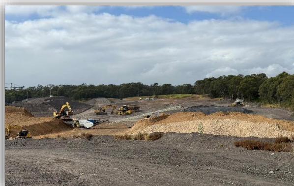
Image 6: Horsley Park Site Works
