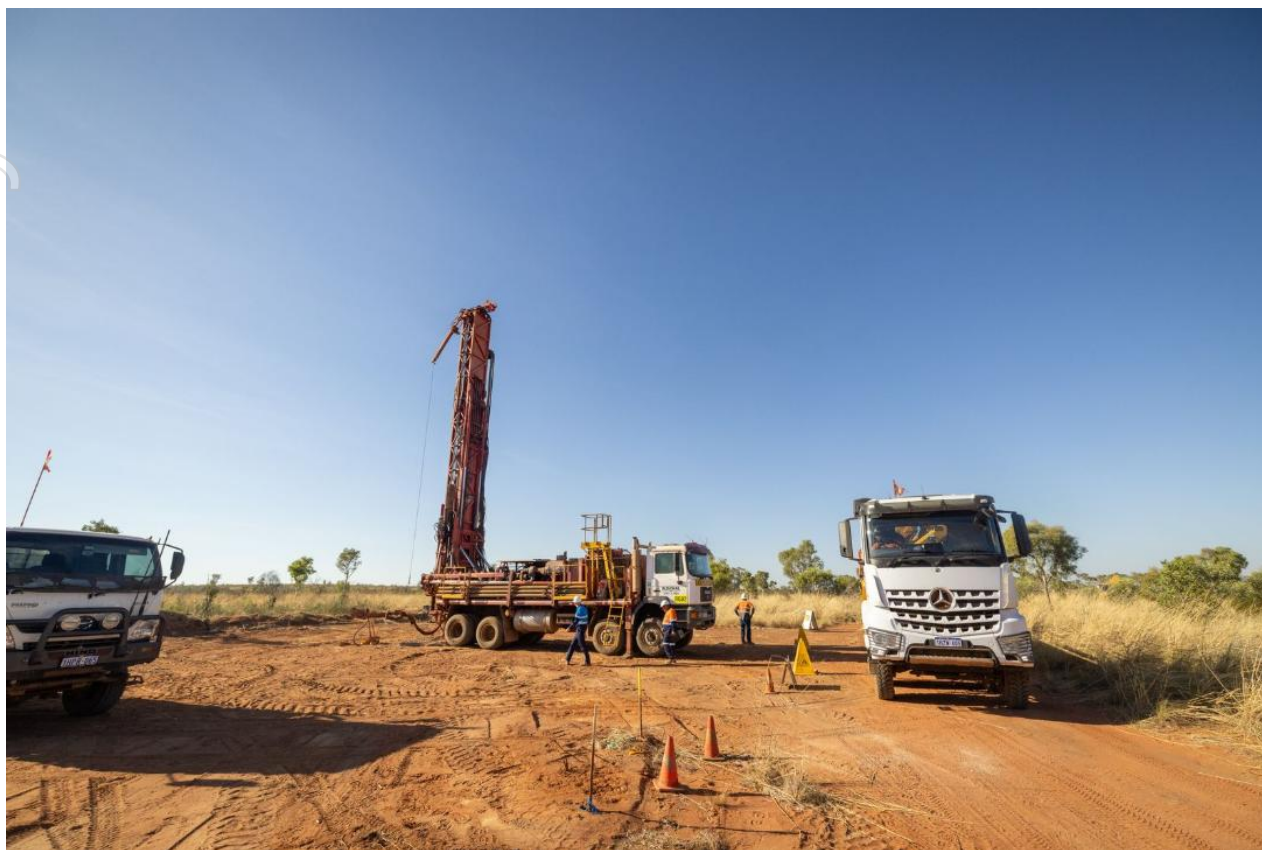
Figure 6 – Construction of water production bores
