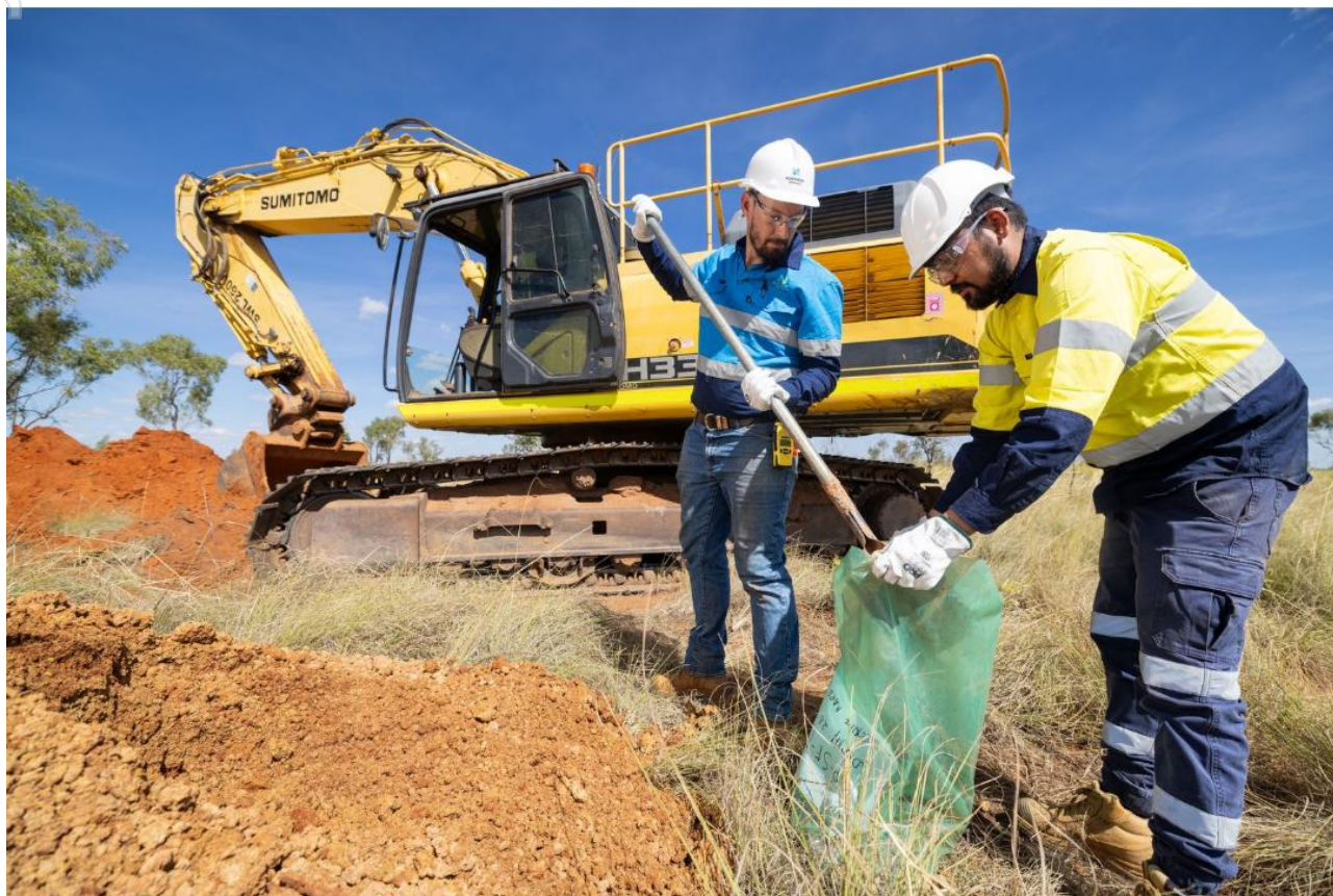
Figure 5 – Test pitting for input into engineering designs
