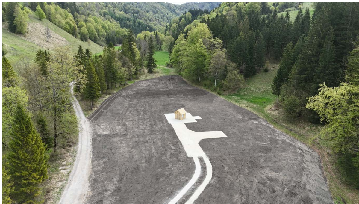
Welchau 1 drilling site area after partial recultivation
