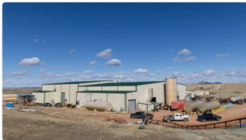
Central Processing Plant (Phase I & II)
