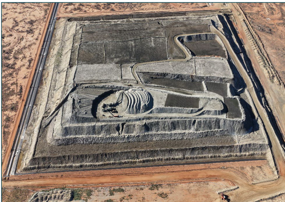
Photo 2: Re-crushing circuit in operation in south western corner of final pad lift
