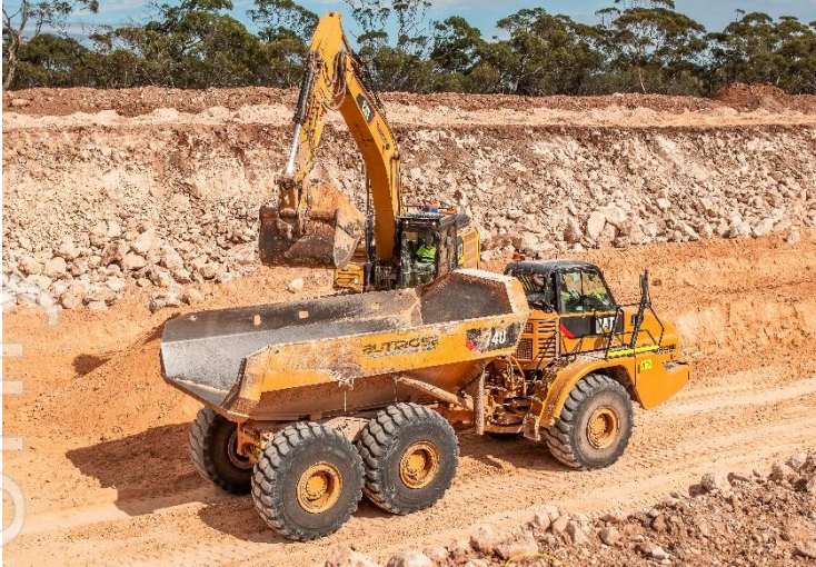
Excavation of the stormwater pond
