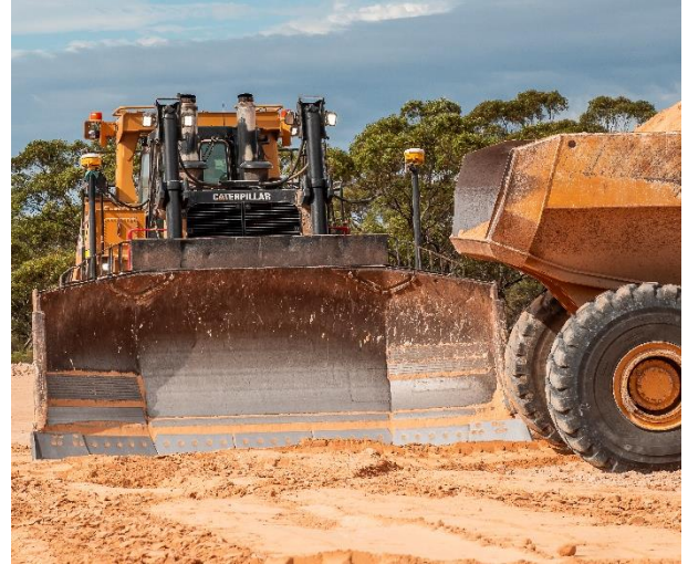
Finalising the processing plant clearance
