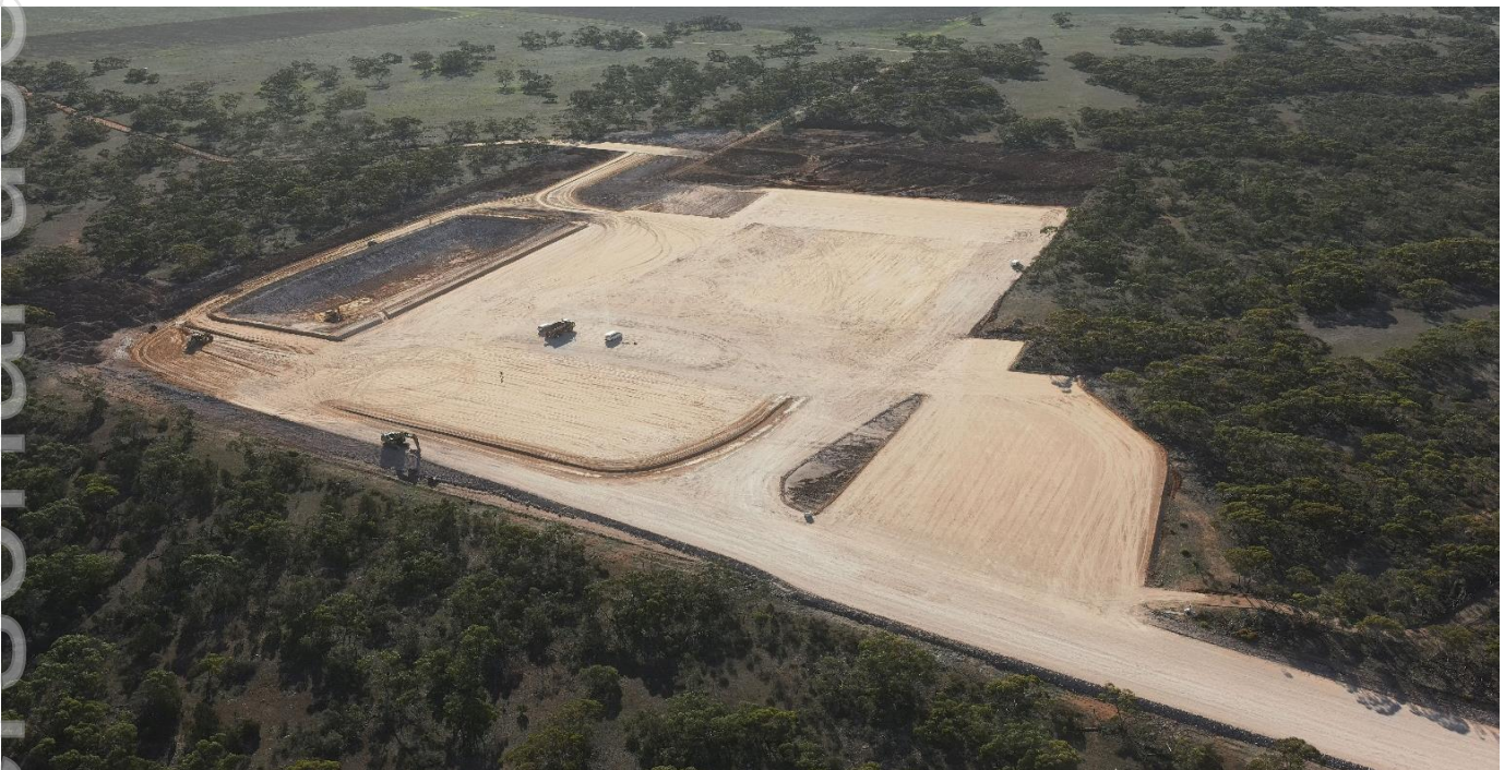
Processing Plant Pad Early Works Construction Completed
