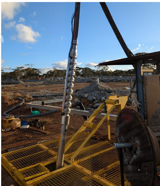
Photo 6 and 7: Dewatering pump being lowered into the shaft and Bore field investigations
