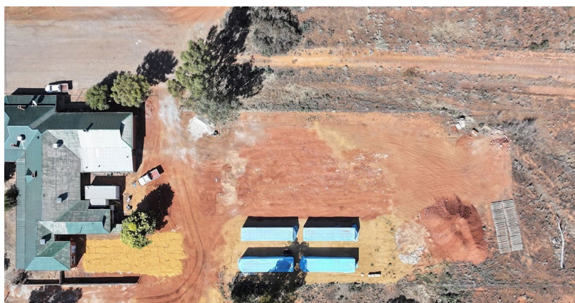
Photo 8: Rear of tavern, location of new camp install to incorporate all 10 donga blocks
