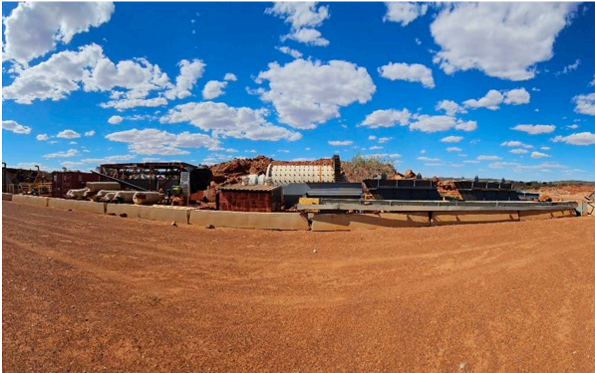
Photo 2: Ball Mill and associated plant
