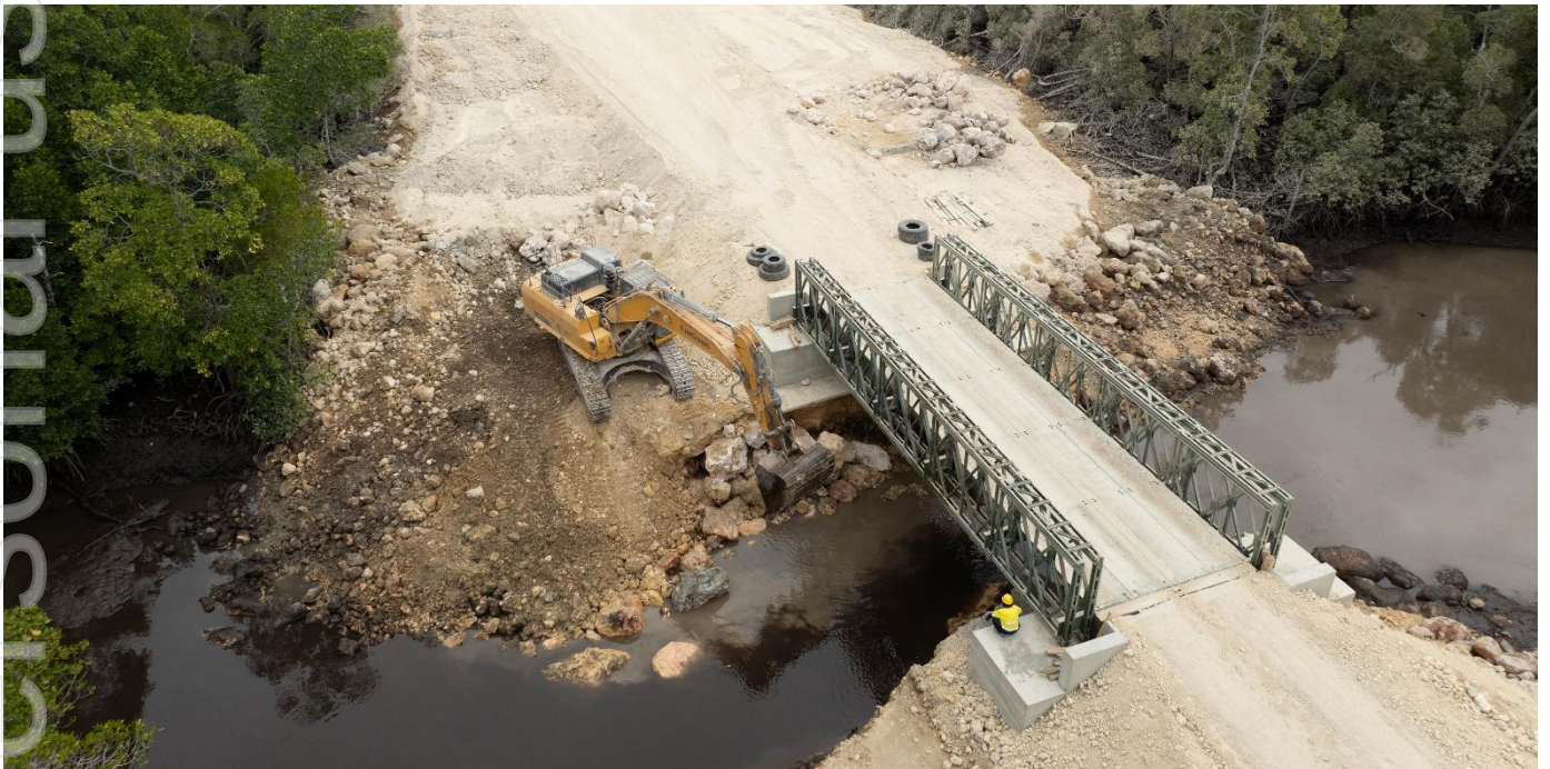
Image: Completed installation of the GEVA Bailey bridge
