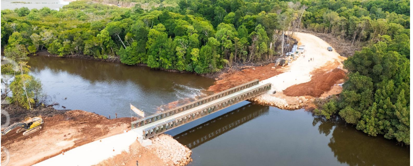
Image: Completed installation of the IBIRI Bailey bridge
