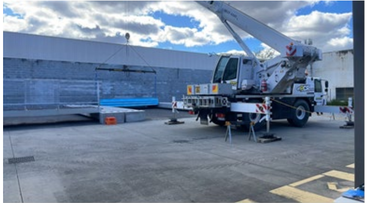
Image 2: Crane ready for module unpacking sequence
