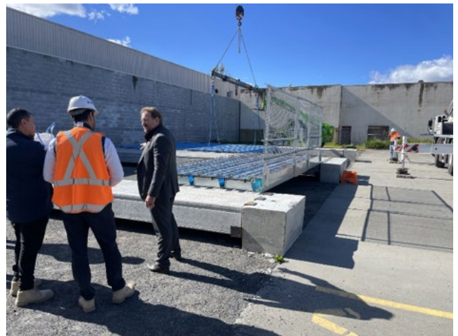
Image 1: Front: Prefabricated module Back: Assembly demonstration
