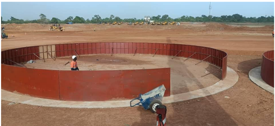
Photo 1 & 2: Process Plant Area at the Kobada Gold Project CIL Tanks - ring beam construction commenced with setting up of formwork
