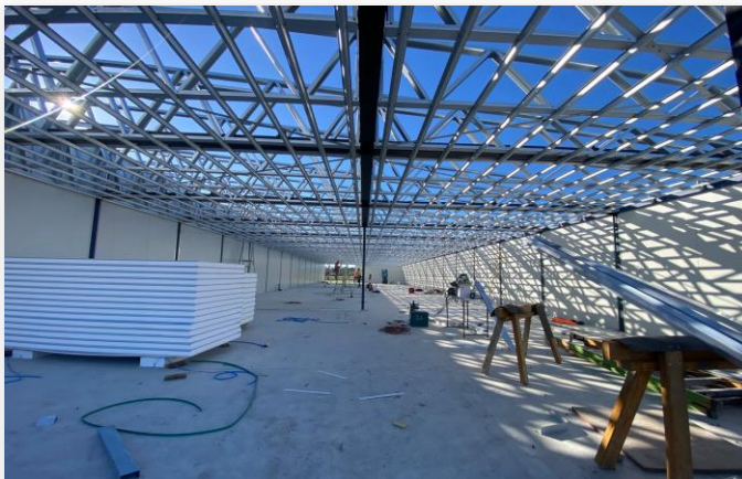
Progress at permanent Mine Services Area (MSA)
