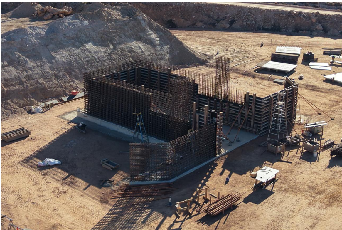
Figure 2 – Primary Crusher steelwork
