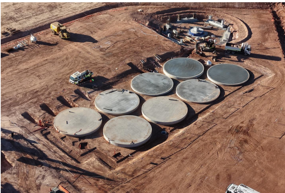
Figure 4 – CIL circuit and tailings thickener footings
