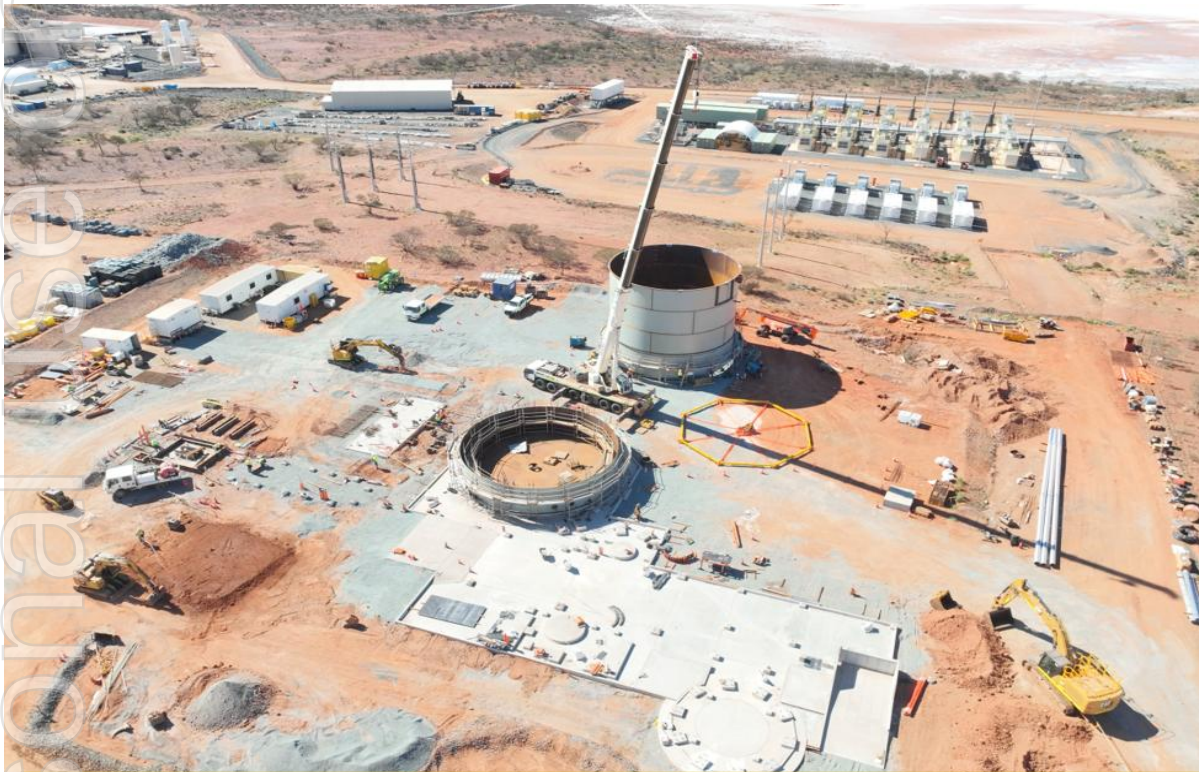
Paste plant Construction on 24 July 2026
