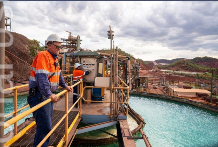
Processing plant & surface infrastructure
