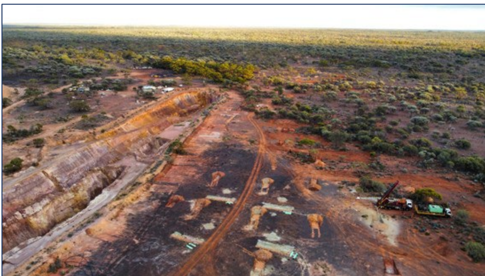
Figure 1: Zelica's pre-existing trial open pit at the Zelica Gold Project, Western Australia
