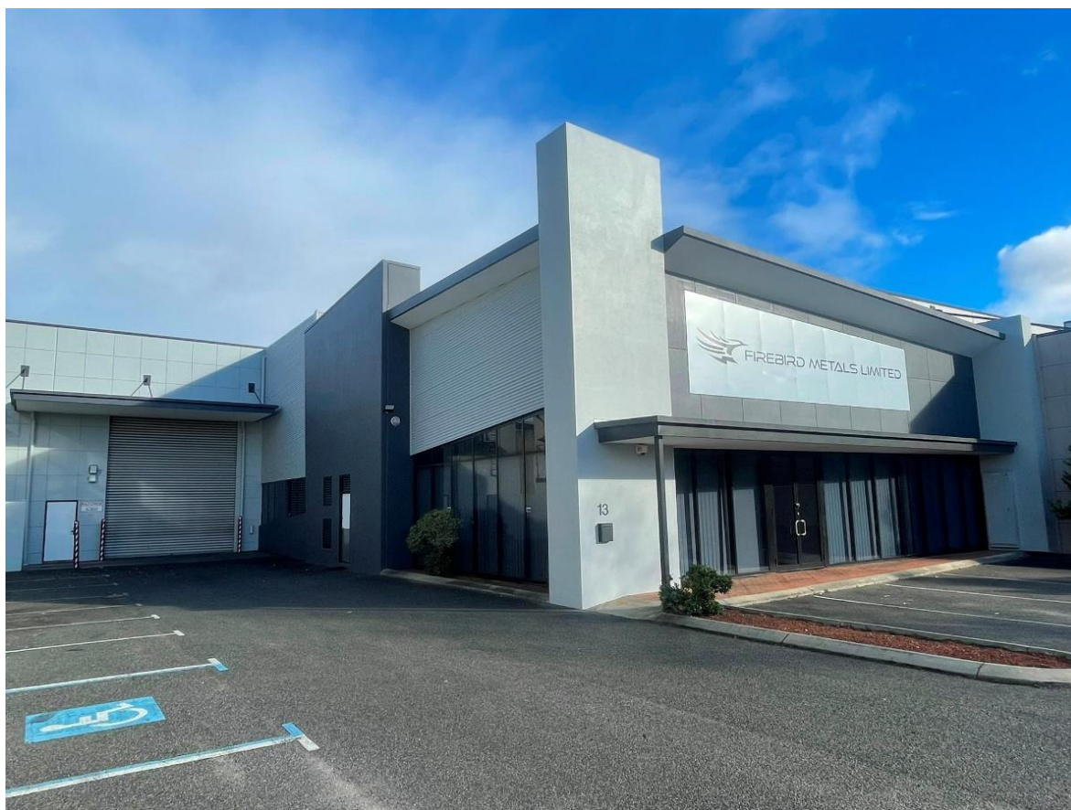
Figure 1. Firebird's new Australian Demonstration Plant site at Osborne Park, Western Australia.
