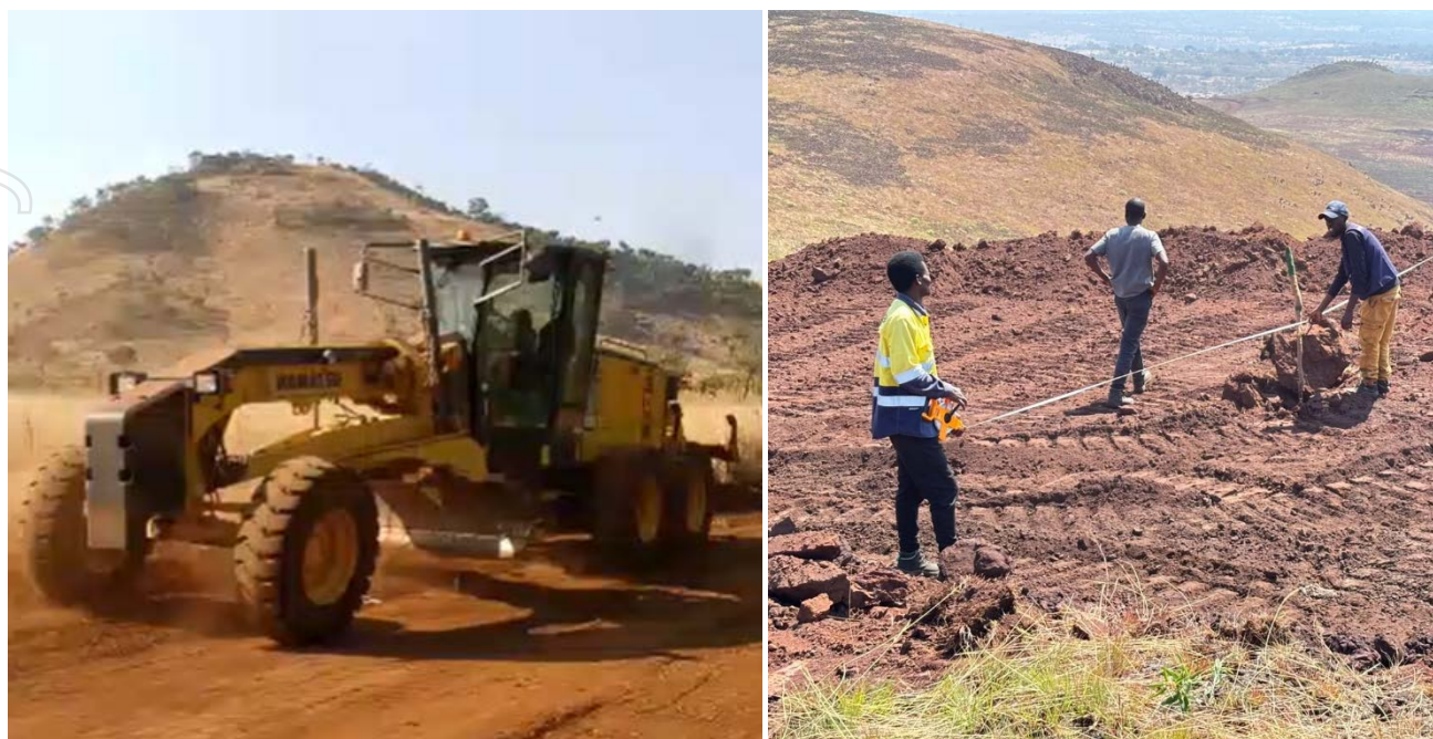
Figure 2 – Road access and drill pad preparations underway at Bailundo
