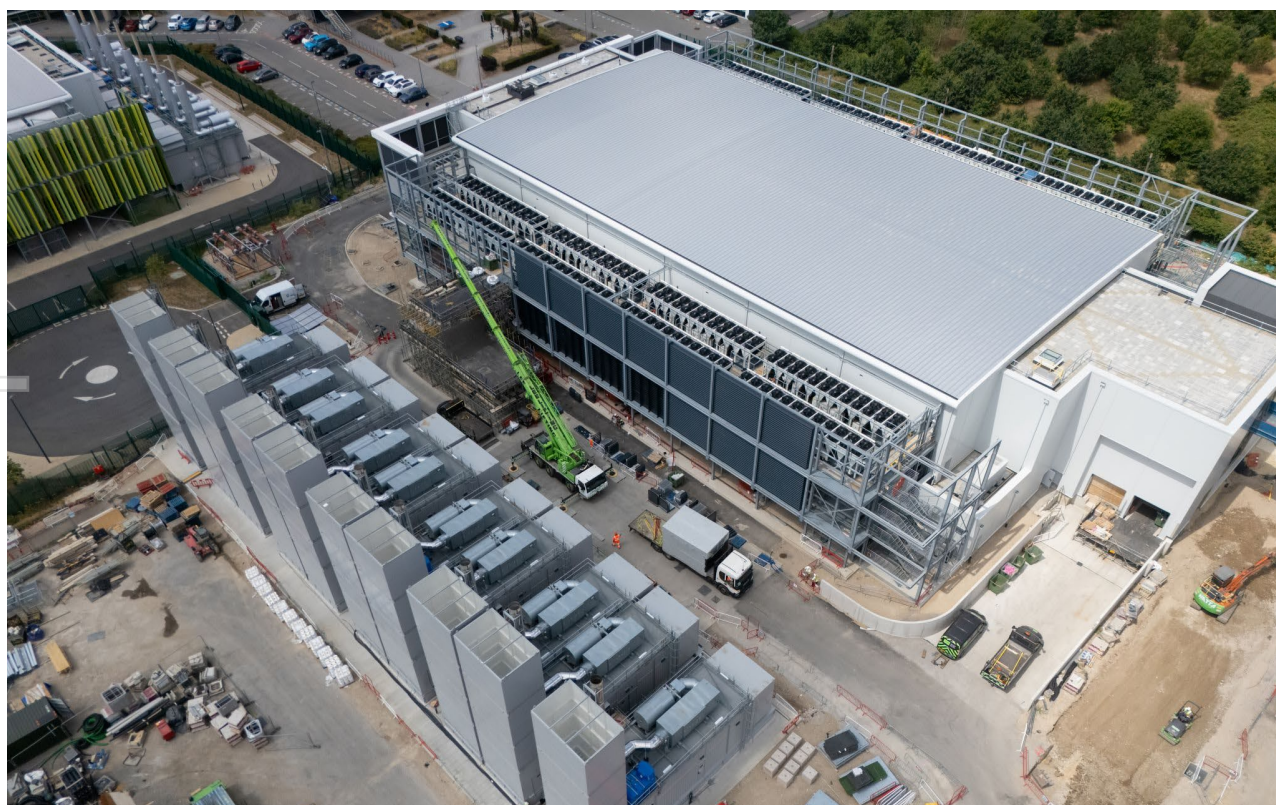
Construction underway at Kao’s KLON-03 facility
