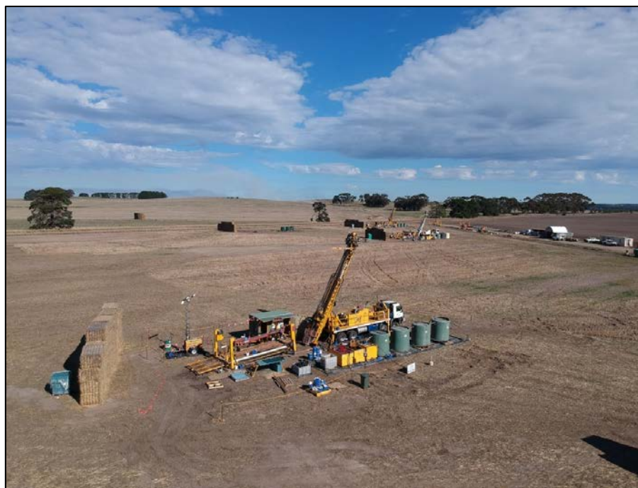
Photo 1. Stavely Project drill-out.
