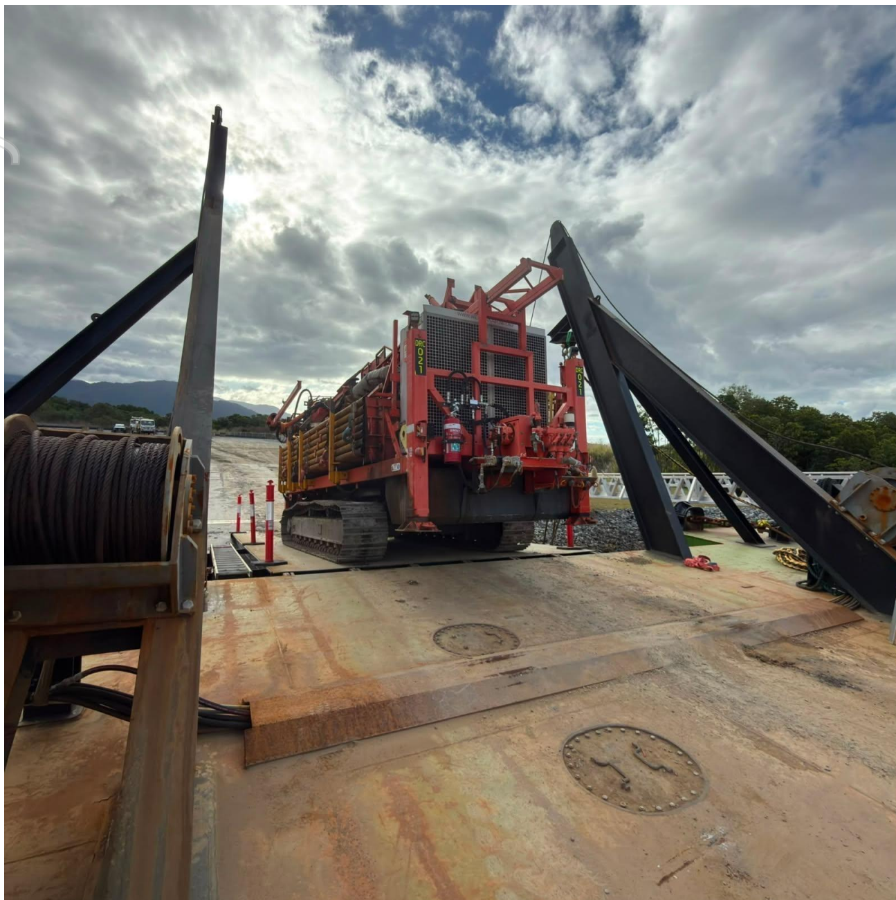
Figure 1. The dual-purpose, track-mounted drill rig being loaded onto the barge in Cairns last week.
