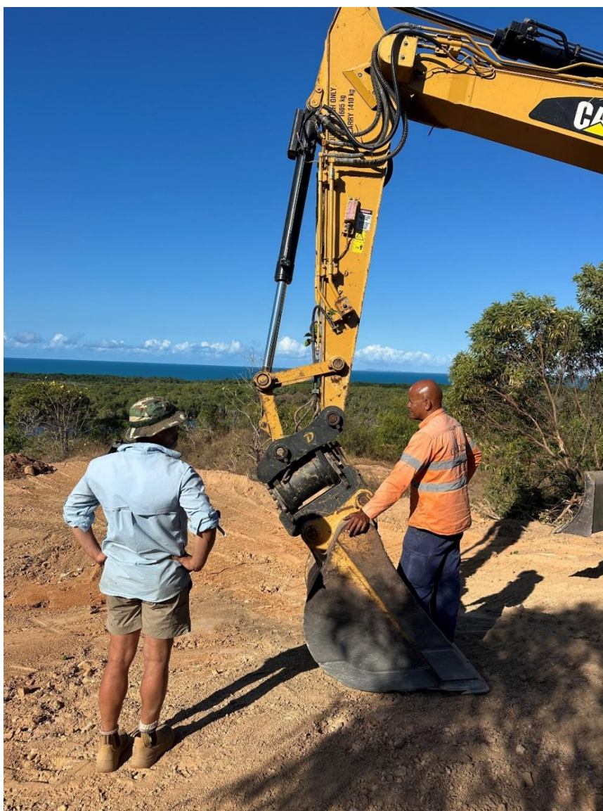
Figure 2. Preparation of drill pads at the Horn Island Gold Project.
