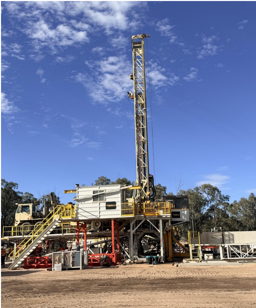
Image 2: Silver City Rig #34 preparing to commence operations on Venus-2H
