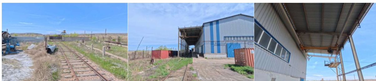
Picture 6. Rail sliding and rail car unloading infrastructure at the SARECO Facility
