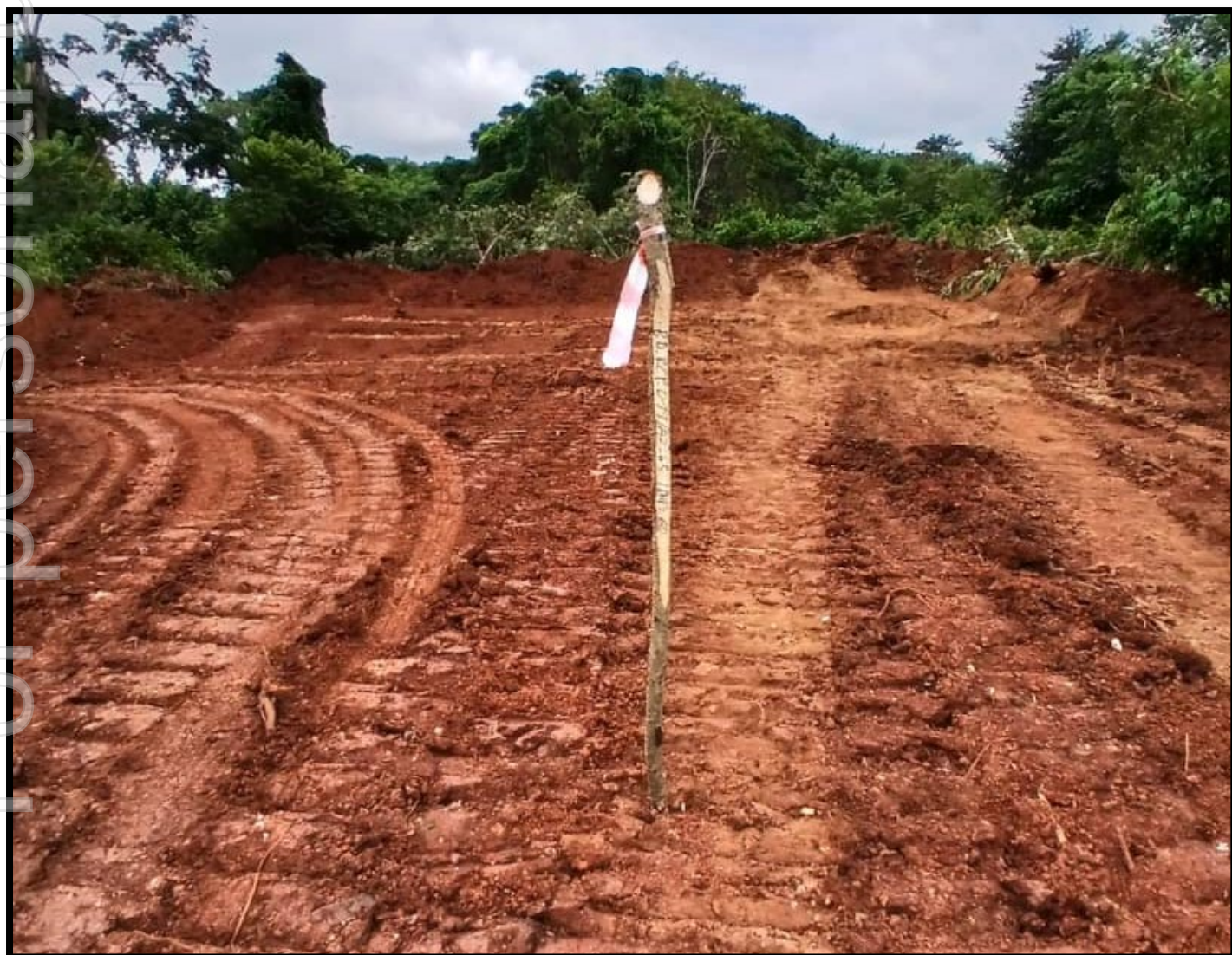
Figure 3. Drill pad preparation complete at Wilfred target.
