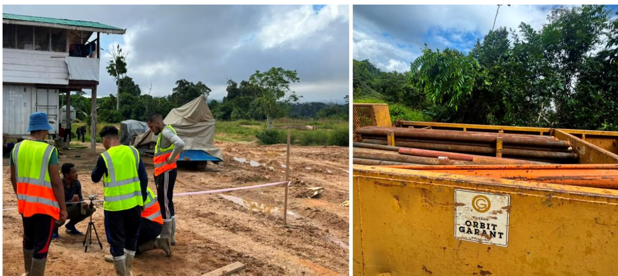
Figure 6: Field crew final simulation for drill rig lining procedures (left) and delivery of diamond drill rods (right).
