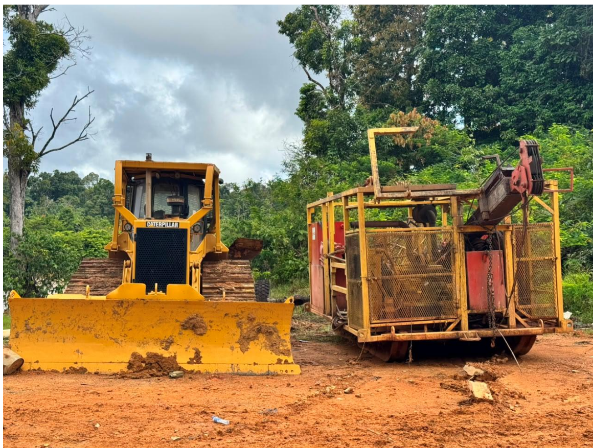
Figure 1: Diamond Drill Rig and Dozer arrival at North Peters.
