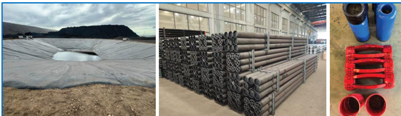
Left: Water pond maintenance completed in July. Middle and Right: Long lead items manufactured and ready for shipment to the Pilot Well Project.
