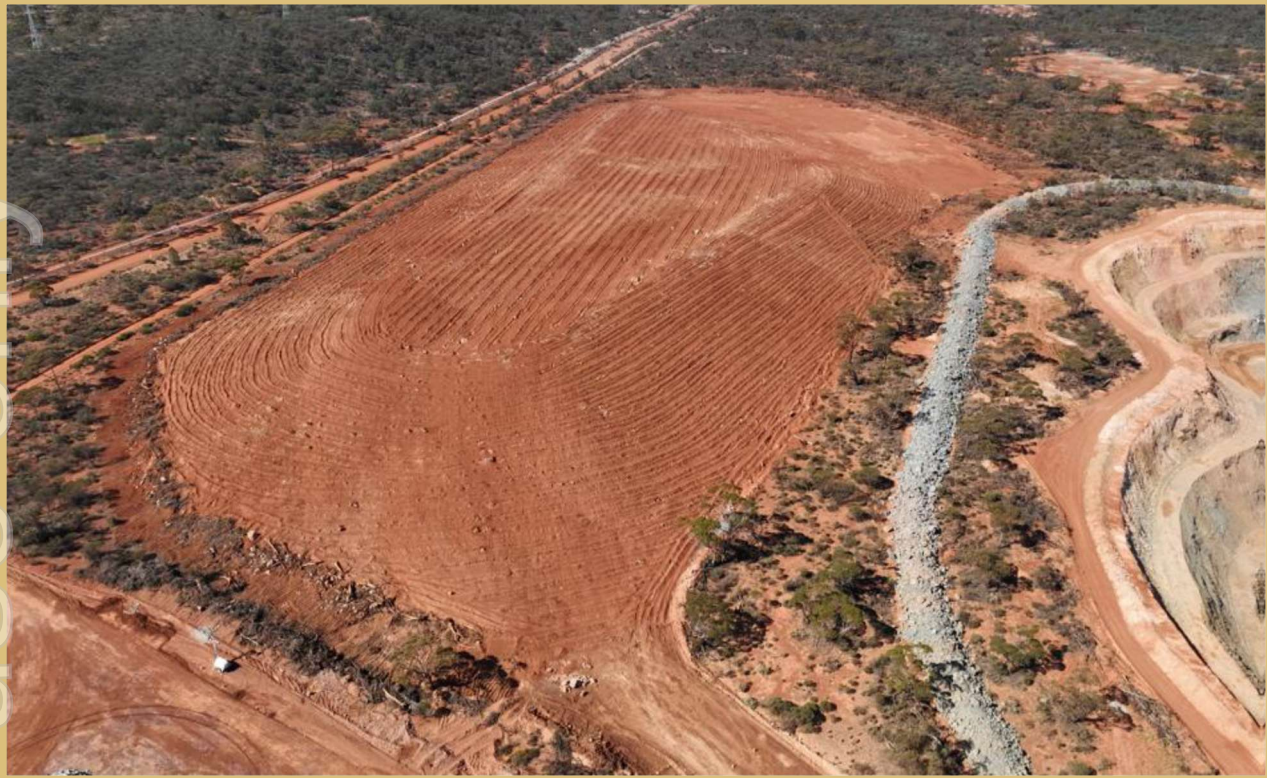
Figure 4: Rehabilitation of the east waste dump is complete.
