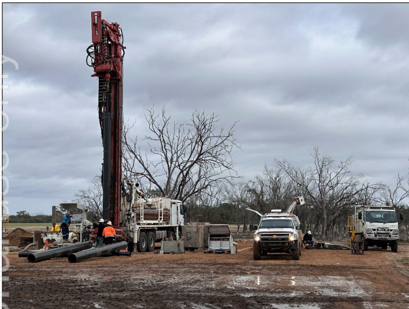
Water bore drilling and bore development at the Gillingarra borefield
