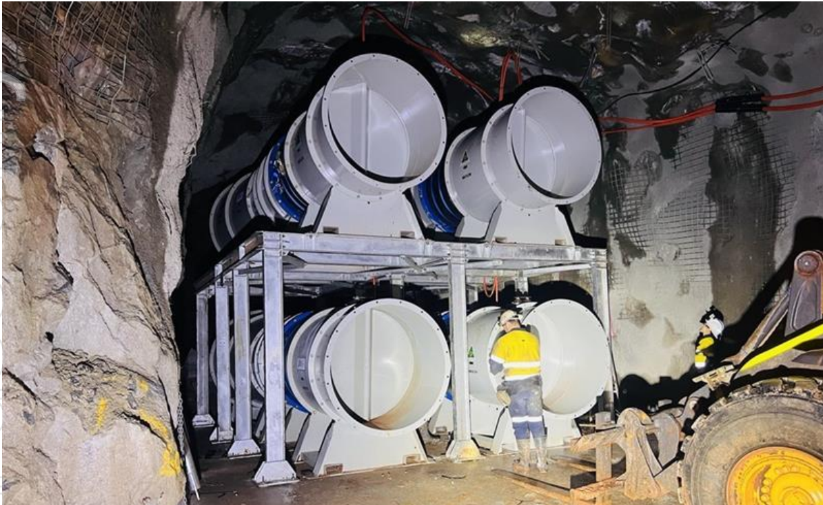
Figure 9 – Installing primary ventilation fans in United North
