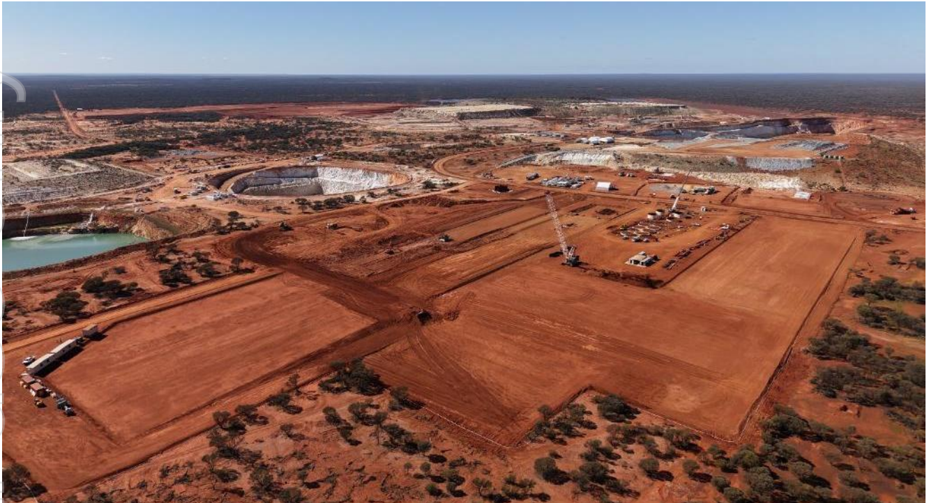
Figure 5 – View of North-West, looking South-East, power station lower left corner
