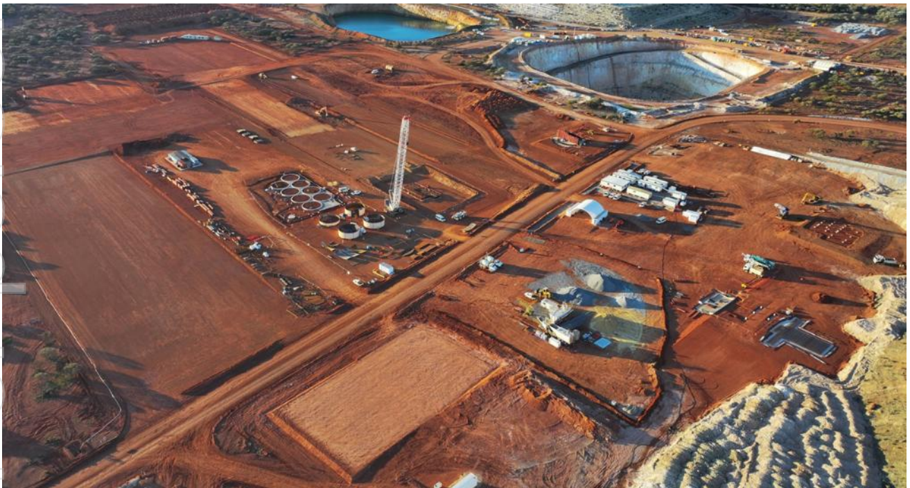
Figure 7 – Mill construction at Youanmi
