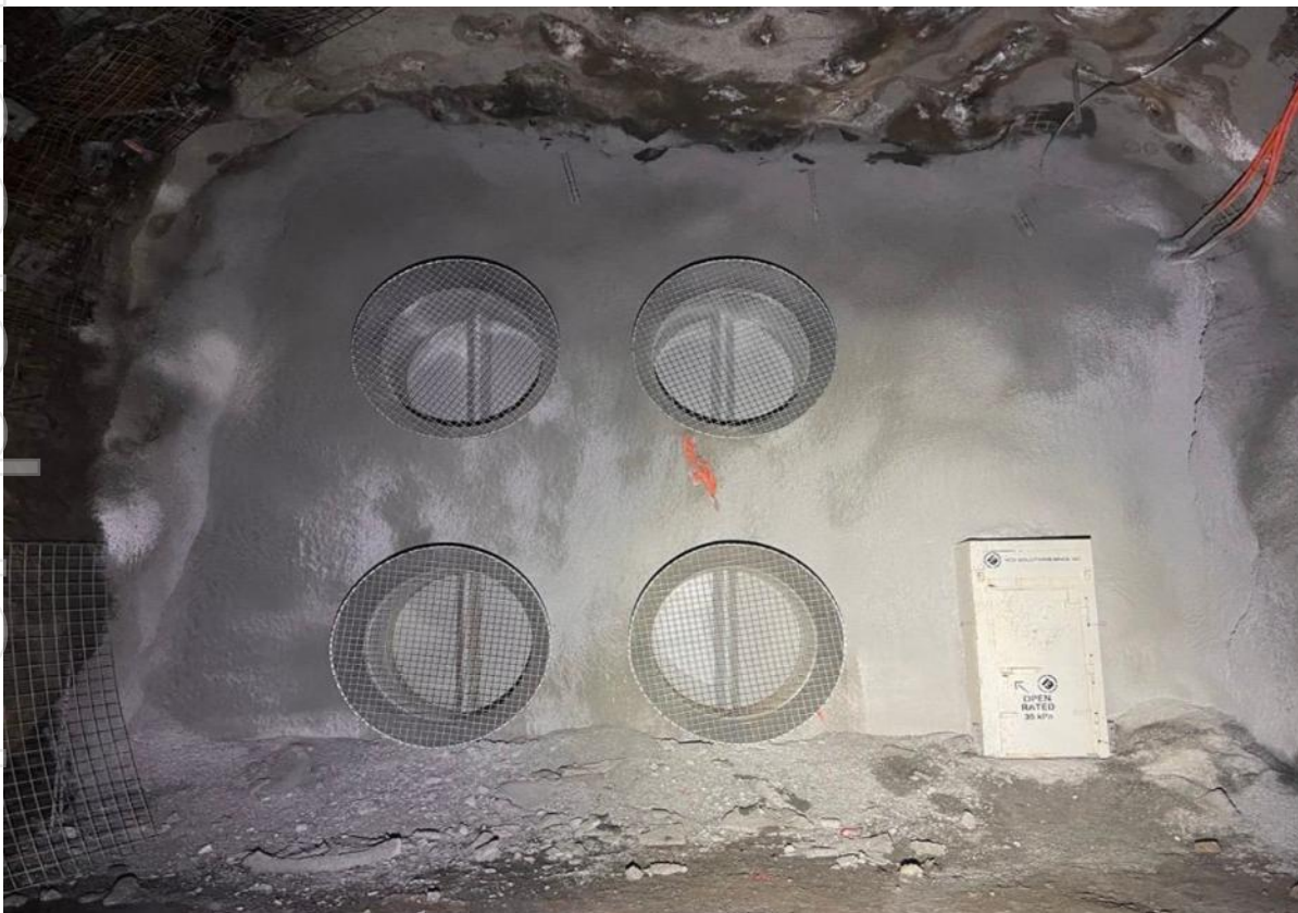
Figure 10 – Installing primary ventilation fans in United North
