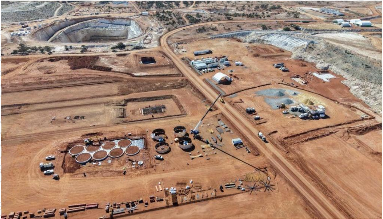
Figure 6 – Progress of construction on site
